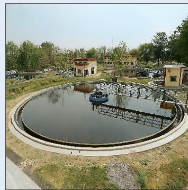
Treatment Plant, Allahabad
