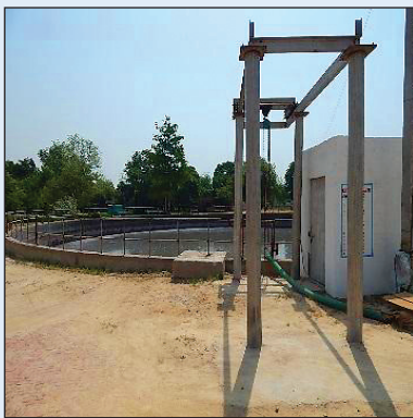
Treatment Plant, Kanpur
