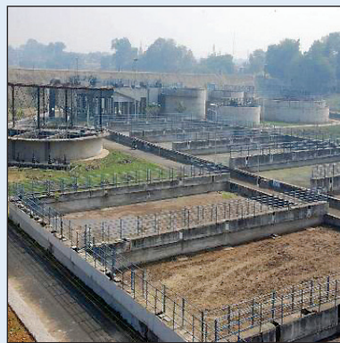
Treatment Plant, Varanasi
