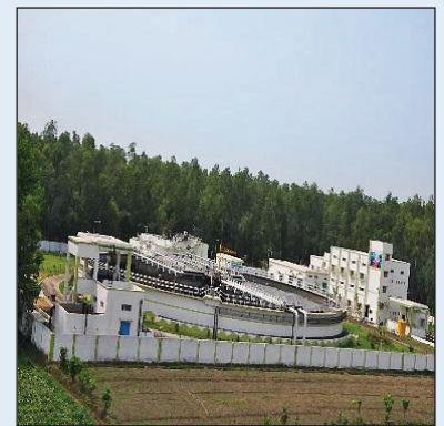
Treatment Plant, Haridwar
